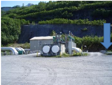
Looking south (uphill)
